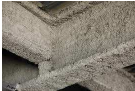
component with spayed asbestos
